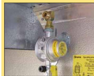
Truma Regulator already supplied with a 90 degree elbow fitted close to a reinforcing strut on the left
