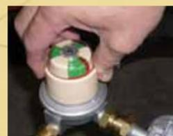
The window will now change to GREEN. Now replace the empty cylinder and open the cylinder valve ready for use.
