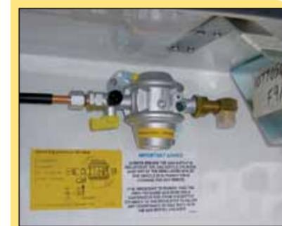
Truma Regulator already supplied with a 90 degree elbow fitted on its side close to a reinforcing strut
