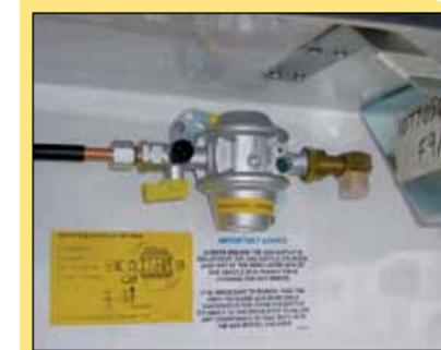
Truma Regulator already supplied with a 90 degree elbow fitted on its side close to a reinforcing strut
