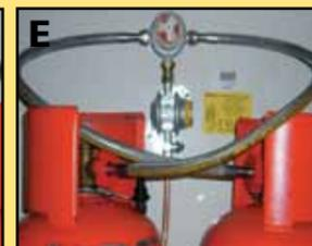
Picture shows a Truma regulator upgraded to an Auto changeover with a 01-1755 and using two propane 0.75 meter Stainless hoses. Note how the hoses cross preventing unnecessary kinking and twisting.
